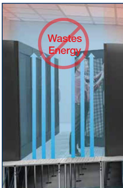
Typical hot aisle/cold aisle layouts have a significant amount of mixing reducing capacity and efficiency.
