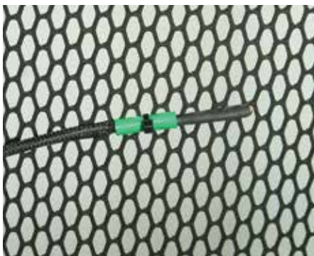
Temperature probes are mounted to the face of the rack
