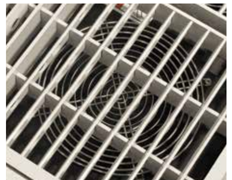
PowerAire fans should only be installed under DirectAire panels to keep the air directed toward the equipment.
