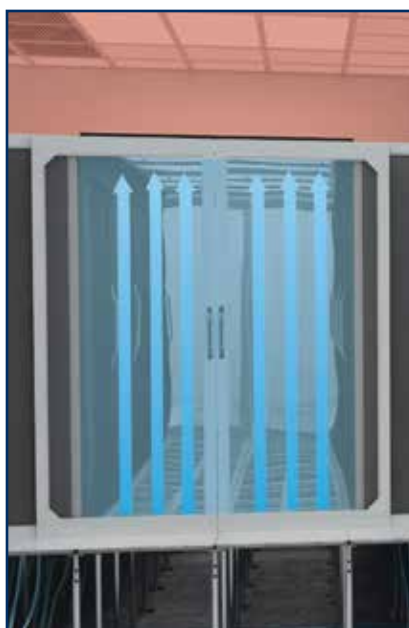
Physical containment can be applied using legacy products to ensure maximum airflow to the racks.
